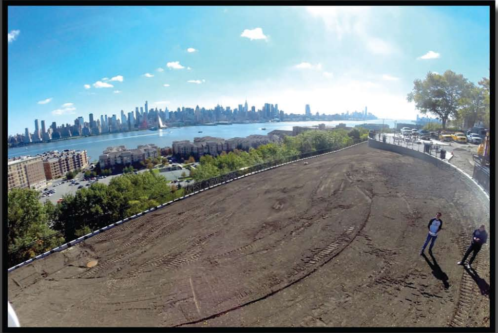
Overlook Fence West New York, NJ
