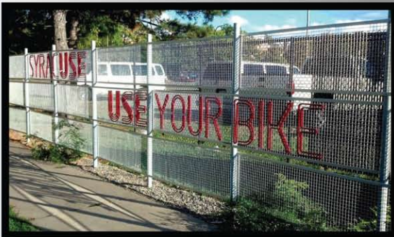
Decorative Urban Park Fence Syracuse, NY
