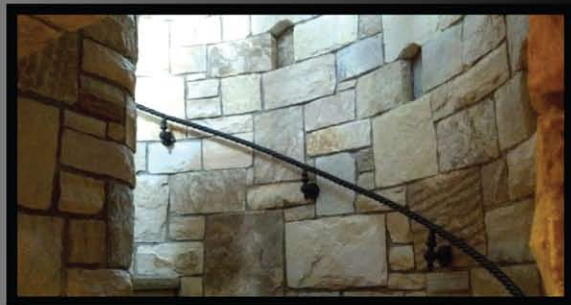
Residential Construction Stairwell Vestal, NY
