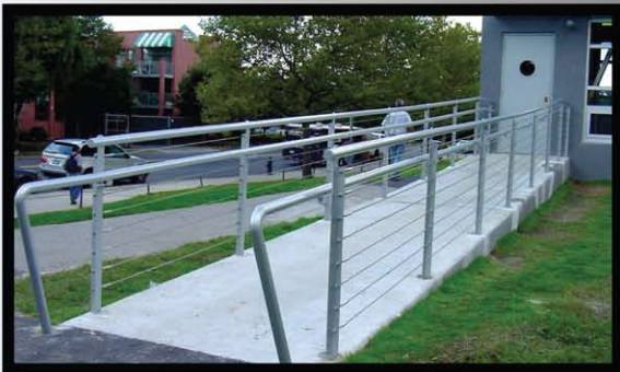
Pedestrian Railings Starlet City, Brooklyn
