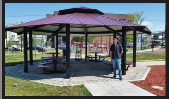
Gazebo Shelter Elizabeth, NJ
