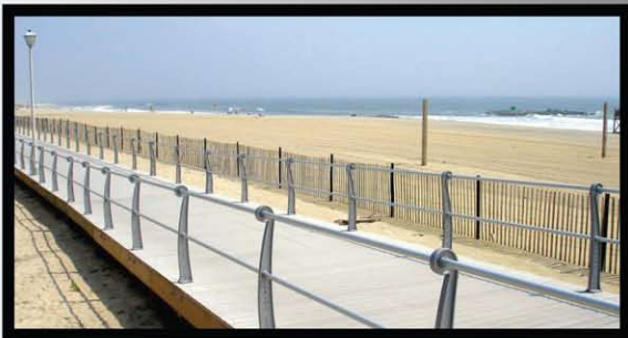
Boardwalk Posts and Handrails Spring Lake, NJ
